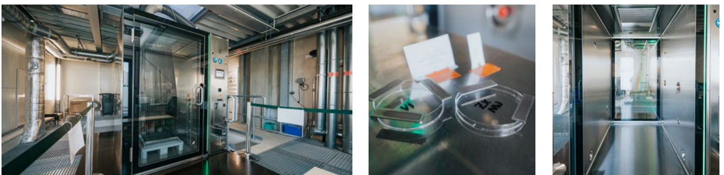
Fig. 4: IDT Biologika is working on the constant optimisation of gassing with the H 2 O 2 -airlock from Ortner Reinraumtechnik GmbH .
